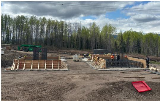
The project's second phase is nearing completion as construction continues in building concrete foundations to support the future substation. Beginning in April, 2024, this phase will be completed by the end of June.
